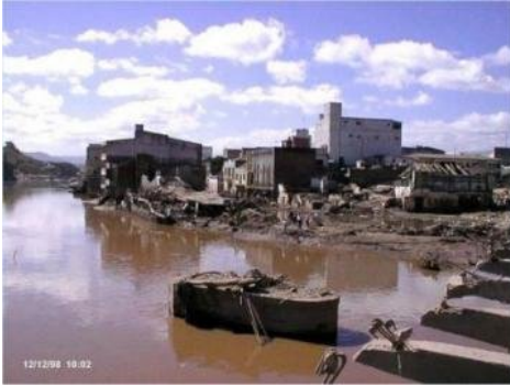
This image shows damage in Tegucigalpa, Honduras caused by Hurricane Mitch in October 1998.
